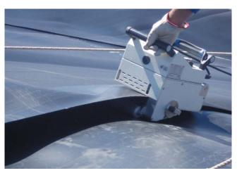
A **HÜRNER** wedge welder HWW 1000 joints a 2.5 mm PE-HD surface lining.
